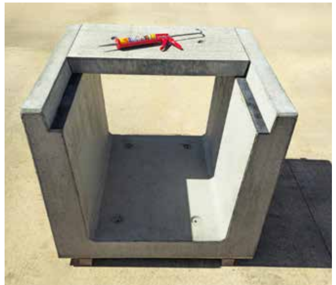
6. Position troughs and where required, apply polyurethane sealant between units.
