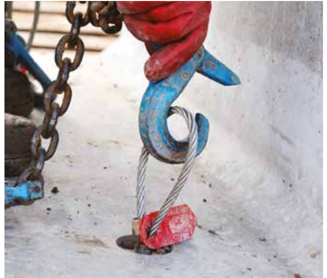
2. Attach lifting chains to all four lifting loops.
