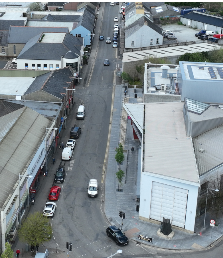
Strabane Library Footpath - Pre Works - April 2026
