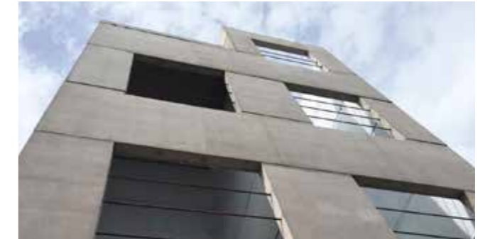
SINGLE LIFT SHAFT
