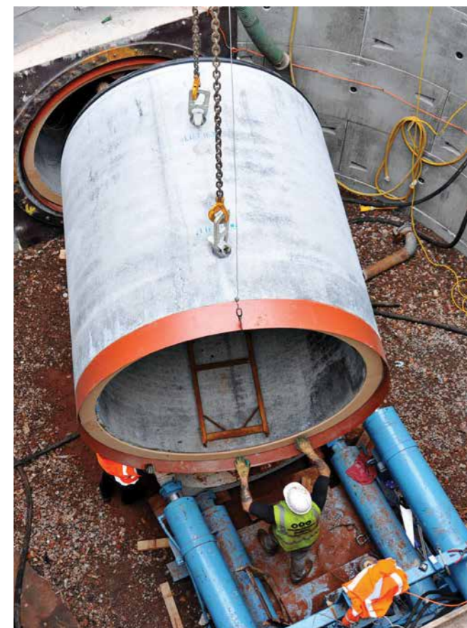
Typical position of jacks relative to pipe wall
