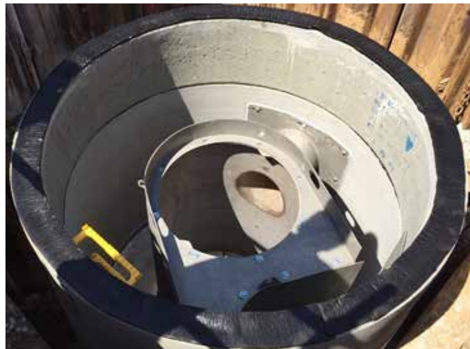
Figure 12 - Main unit with butyl rubber seal installed, ready for cover/access assembly configuration
