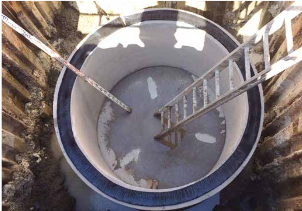
Figure 7 - Butyl rubber seal installed and utility lifting anchors filled
