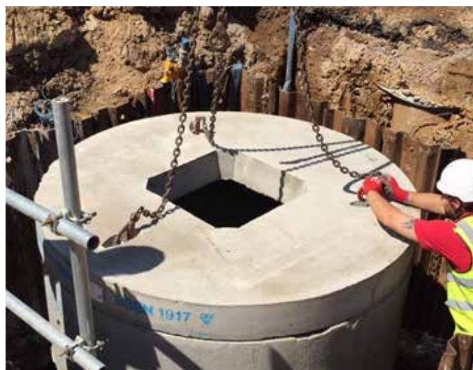
Figure 15 - Site image of cover slab lifting and placement
