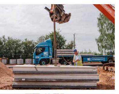
Civil engineer and ground worker Friel Construction, the contractor responsible for drainage, roads and foundation construction to ground floor level, is utilising the brand new Thermabeam flooring system on one of the plots as an initial trial, in support of FP McCann's development of the innovative alternative to traditional solid slab floorina.
