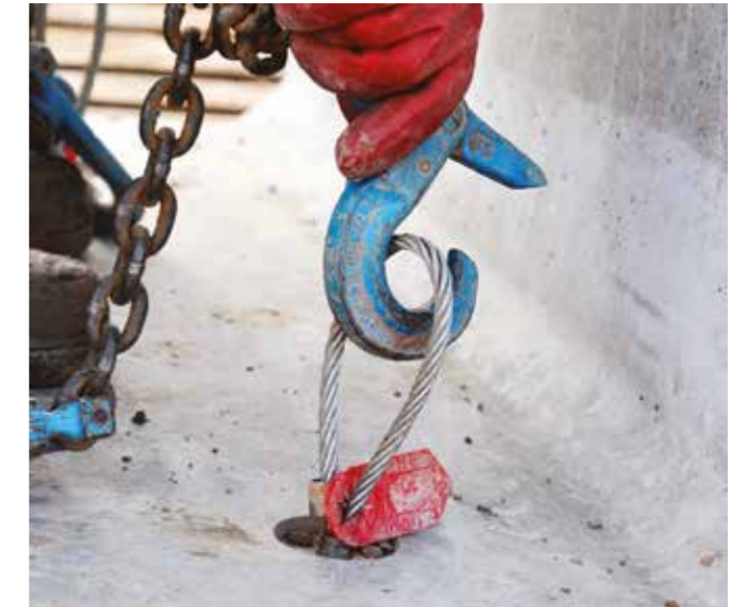
2. Attach lifting chains to all four lifting loops.
