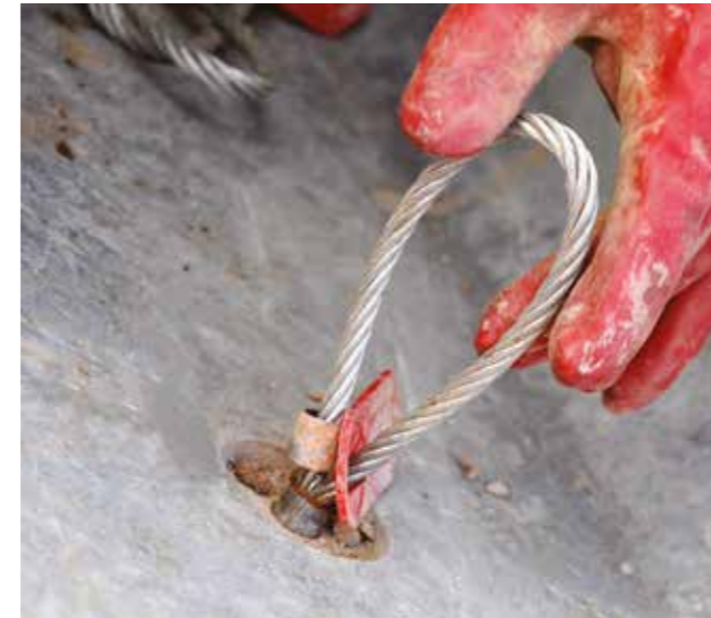
1. Position trough on a level flat area. Fix in lifting loops to each of the four lifting points. Check loops are secure.
