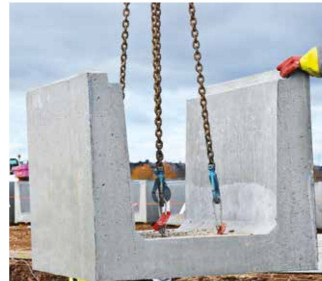
3. Ensure lifting chains are symmetrical then begin lift.
