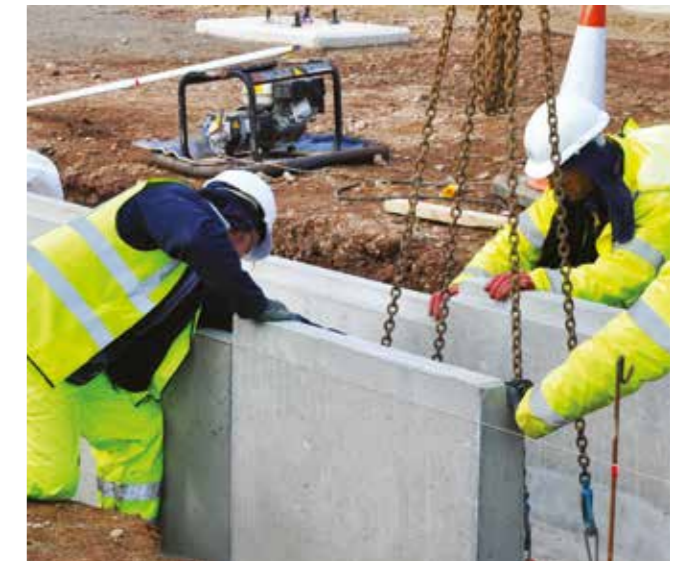
4. Lift slowly and with care, then place trough in position. Ensure trough is in line and level. Then remove lift chains and unscrew lifting loops.
