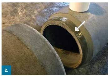
Prior to assembly clean the socket and spigot. Water and mud does not seriously affect the joint, but should be avoided. It is recommended that only a FP McCann approved lubricant is used. Apply lubricant to the spigot end. Take care that lubricant is evenly applied all around the spigot. It is important to lubricate the radius area, as shown by the arrow in the picture. Lubrication is easier with the pipe suspended. Dry jointing can result in severe damage to the seal and pipe.
