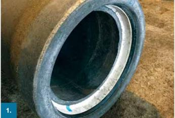
Prior to assembly, inspect the pipes and ensure they are in good condition. The white protective strip in the socket helps to keep the sealing area free from dirt, mud and gravel etc.
