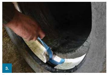
The protective strip is removed prior to jointing. Grip the tab of blue tape and pull towards the pipe centre- not towards the inside or outside. Small parts of the strip can remain in the pipe without affecting the joint performance.
