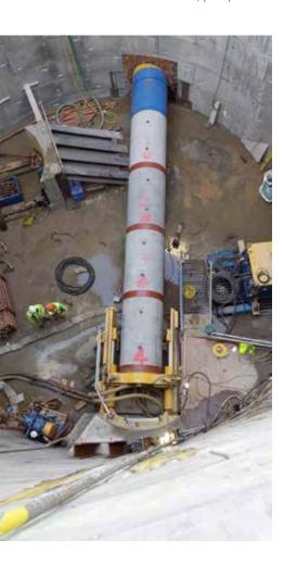
As well as the large 15metre diameter, storage tank capable of holding 1700m3 of storm water, the project involves four drive/reception shafts, 550metres of DN 1200mm and 70 metres of DN 600mm pipe jacked tunnel, also acting as online storage. FP McCann has supplied both the smoothbore precast concrete shaft segments and the jacking pipes to the contract.
