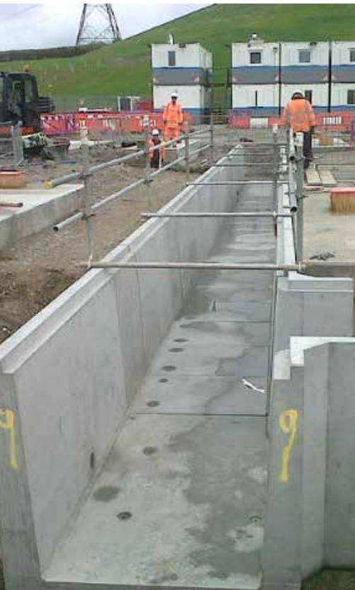
FP McCann's Easi-Duct precast concrete cable troughs are being installed by Morgan Sindall, a main EAC construction partner along with ABB and Atkins. The troughs are to carry high voltage cabling to and from the new gas insulated switch-gear (GIS) substation. The access troughs are buried flush with the surface to protect the power network from accidental or malicious damage, but allow for easy access for maintenance and repair.
