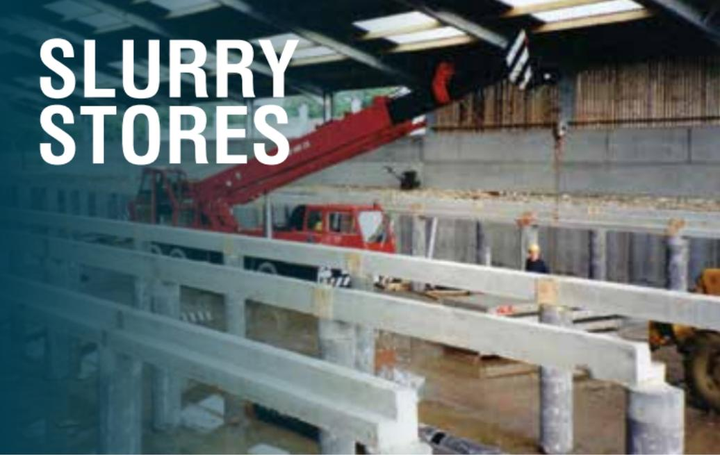
FP McCann's slurry panels are made from high-quality prestressed concrete, designed in accordance with BS 5502.
