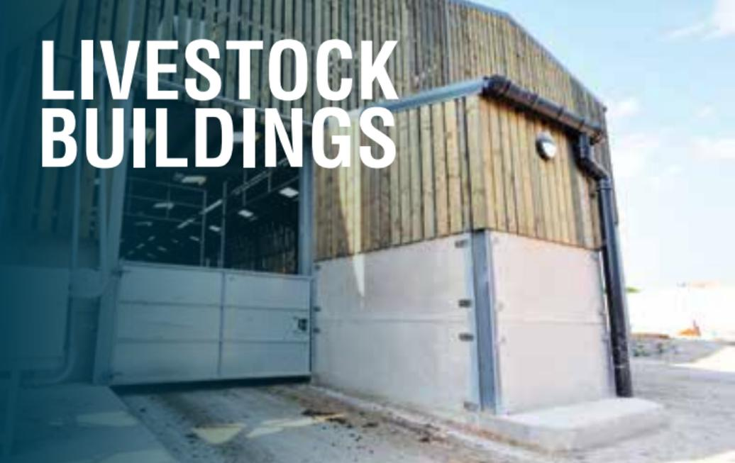
Prestressed concrete panels are an ideal, hygienic solution for containing all types of livestock. The 80mm thick prestressed panels are lightweight and quick to install, providing superior strength to withstanding impact load from livestock. The prestressed manufacturing process provides built-in strength and resilience, whilst using less concrete results in a better engineered and more cost-effective solution.
