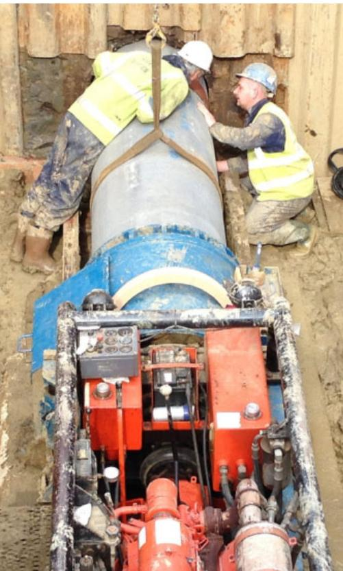
FP McCann supplied DN 600mm precast concrete jacking pipe from its Alnwick facility in Northumberland which was installed using guided auger boring trenchless technology, typically utilised in deep pipeline drives.
