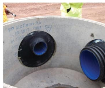
Once pipe is fitted to connector, up to 45° of deflection is possible without breaking the seal.
