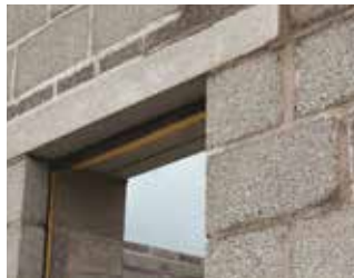
Concrete lintel as used traditionally in construction.
