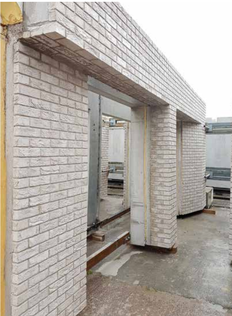
Textured/pattern imprinted cladding panels
