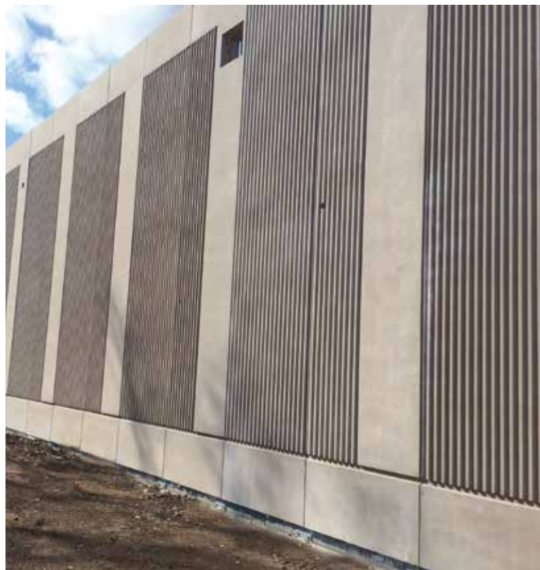
Textured/pattern imprinted cladding panels
