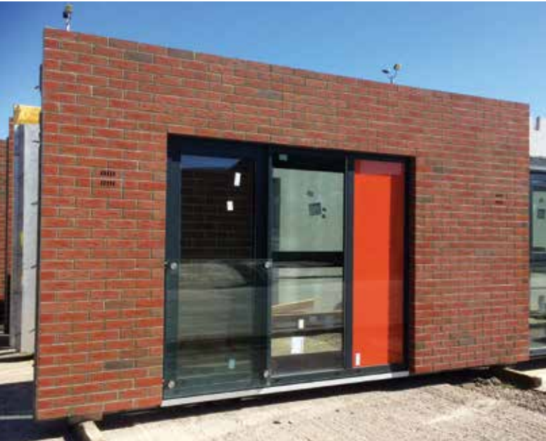
Fully pointed with windows built-in
