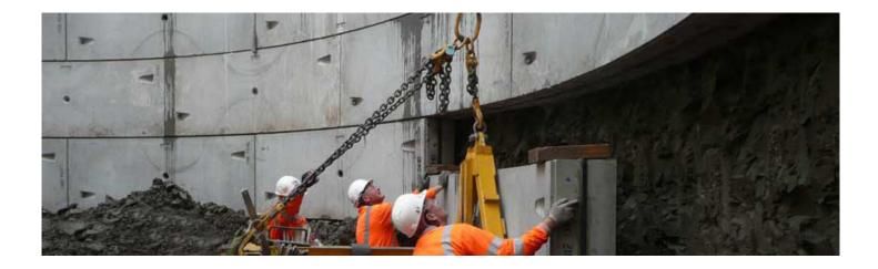
FP McCann manufactures a comprehensive range of smooth shaft segmental rings suitable for underpinning, caisson and chimney construction methods. Factory pre-fitted EPDM rubber gaskets are standard on all segments providing an immediate water-tight seal on construction. Additional to cross joint and circle joint bolting systems, FP McCann offers a safer and more efficient back bolting system for the caisson build method.
