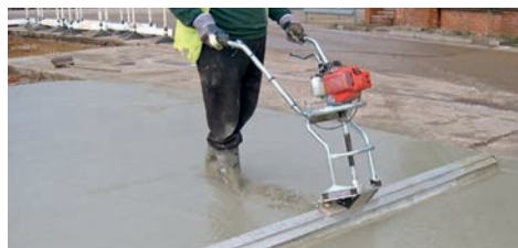
Figure 13. Petrol powered single beam screed
