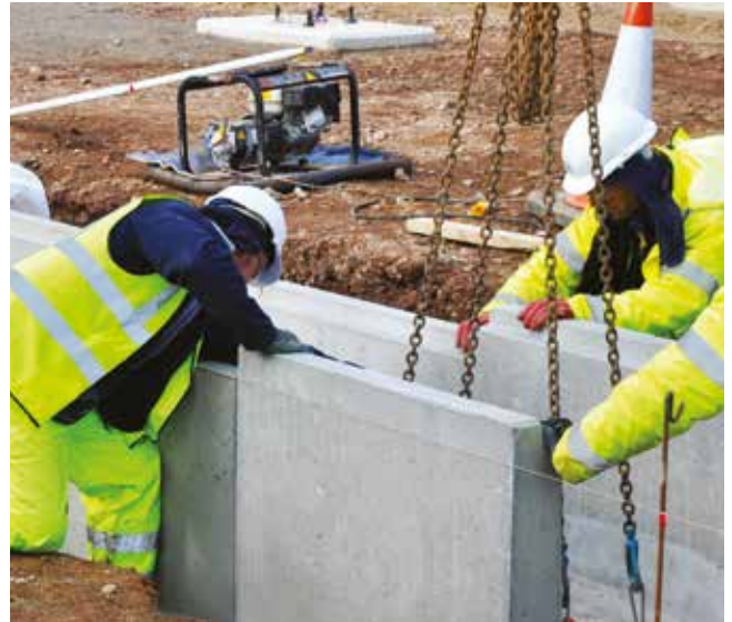
4. Lift slowly and with care, then place trough in position. Ensure trough is in line and level. Then remove lift chains and unscrew lifting loops.
