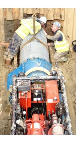
FP McCann supplied DN 600mm precast concrete jacking pipe from its Alnwick facility in Northumberland which was installed using guided auger boring trenchless technology, typically utilised in deep pipeline drives.
