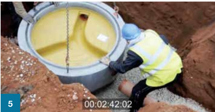
5. Prior to connecting, the pipes are lubricated using an FP McCann approved lubricant. When positioning the base the outlet point is indicated by an embossed arrow.
