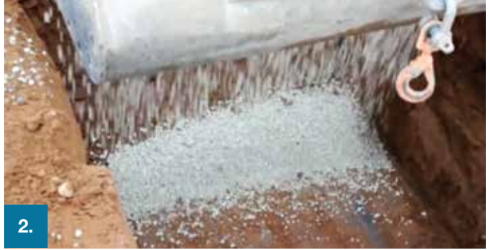
2. Suitable granular material is added.
