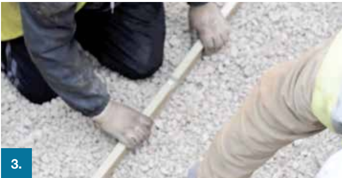
3. Bedding material is compacted and levelled to provide a solid bed.
