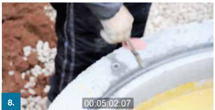
8. Integral lifting loops are then removed from the easi-base unit.
