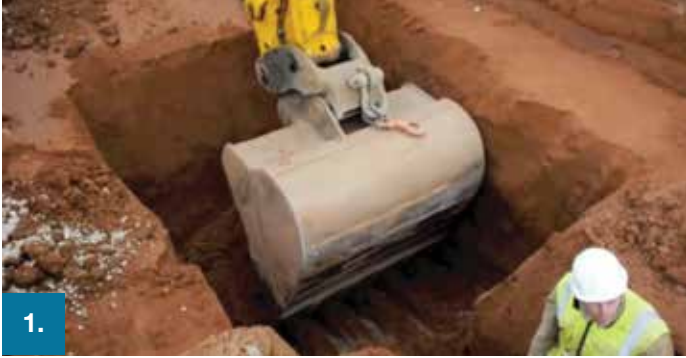
1. The base of the excavation is prepared.
