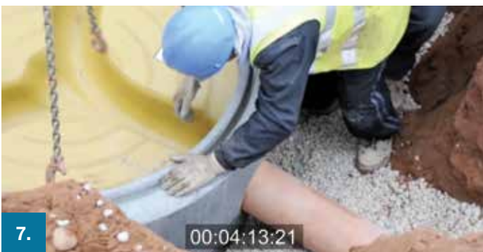
7. A degree of deflection is achievable, this will vary depending on pipe type and size.
