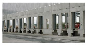
The front, rear, and end side walls are designed to be supported off and are connected to a reinforced structural concrete foundation slab. The foundation slab is to be designed and installed by others to suit the ground conditions and wall loadings.
