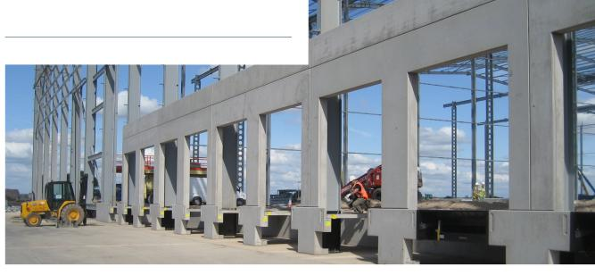
The FP McCann Ltd Single Door Prowall walling system is designed in insulated reinforced precast concrete. The integral insulation will provide an elemental U-value of 0.22 W/m2K. Better U-values can be achieved by increasing insulation size, but this will incur additional costs.
