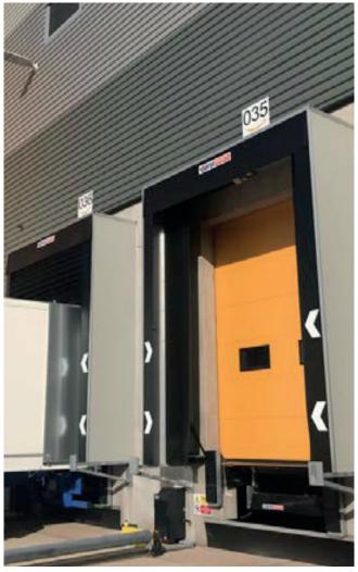
Doors will only require support from the steelwork above the panels, as tracks can be connected directly to the internal face of Prowall. Dock shelters can be externally attached if needed.
