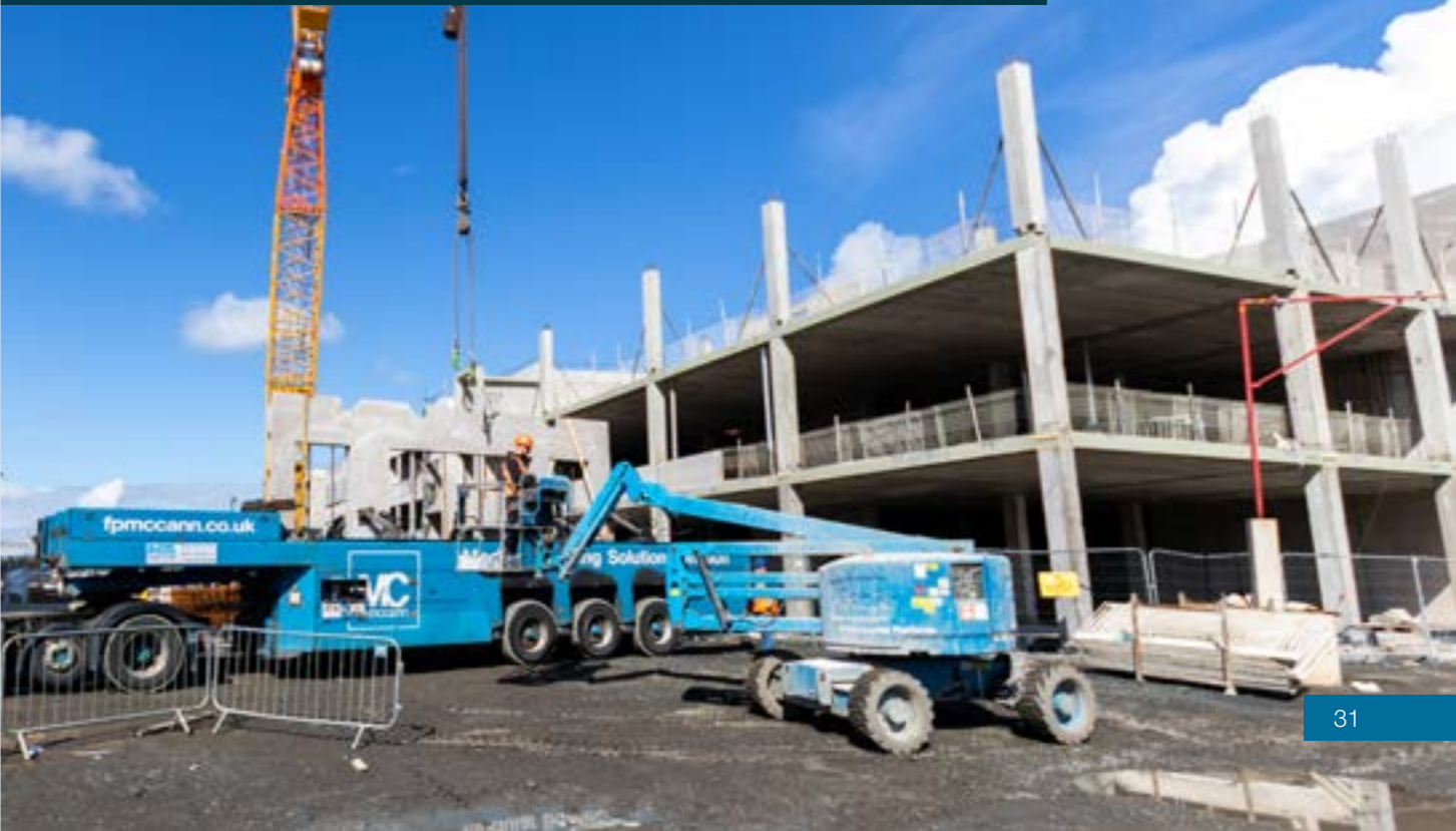
Precast columns, combined with floor sections, allow for efficient construction of the structural frame.
