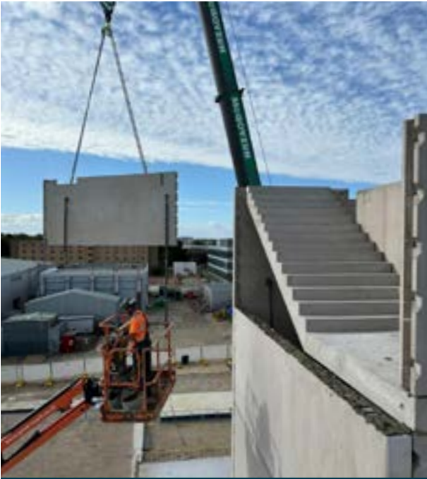
Each stair core section is craned into position with ease.
