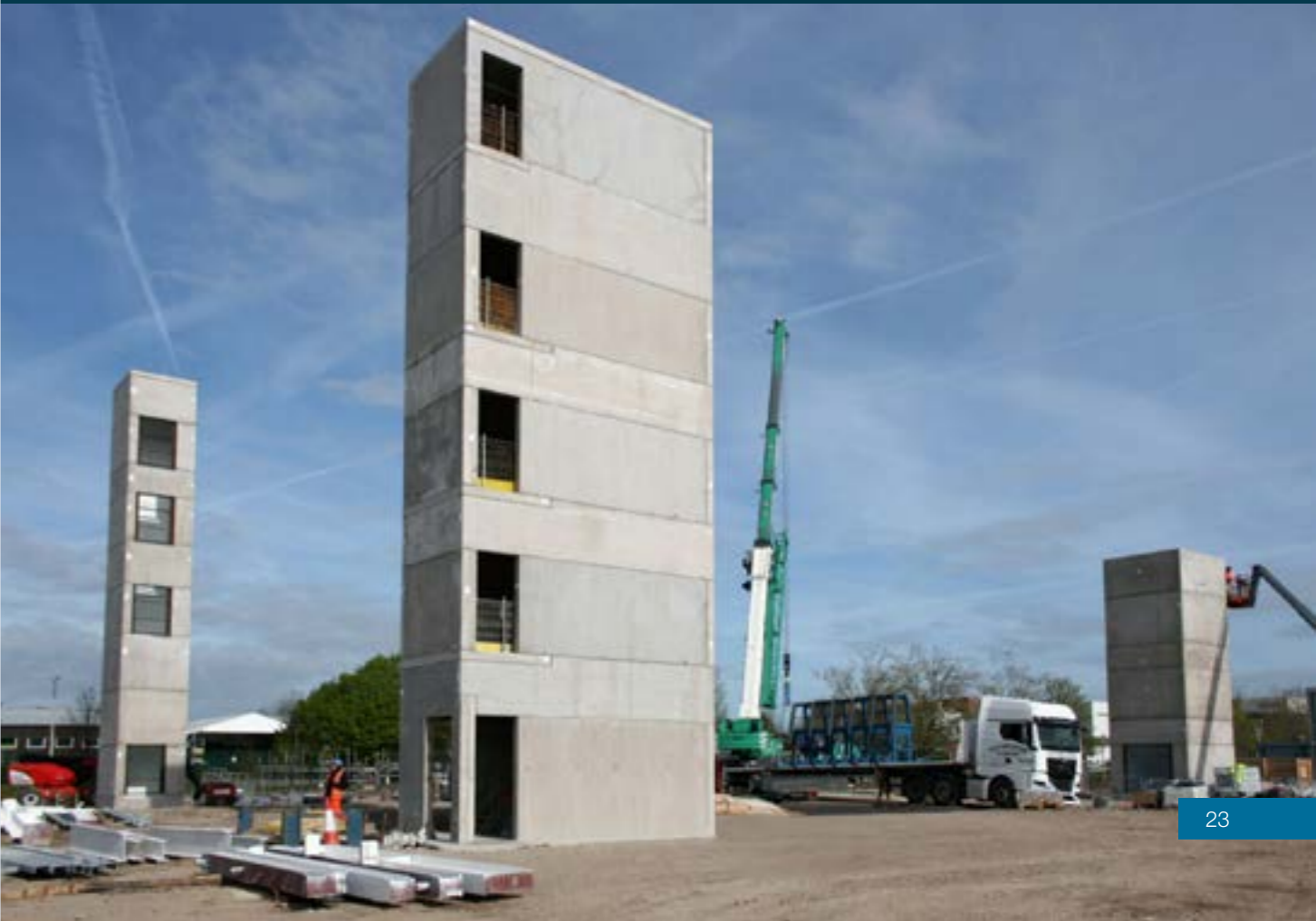
FP McCann's precast lift shafts are constructed in a fraction of the time needed for casting on-site.
