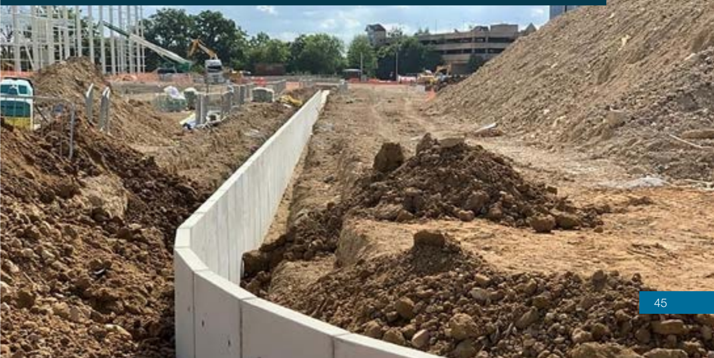
Retaining walls created using FP McCann's precast L-Walls can be designed to meet a wide variety of site requirements.
