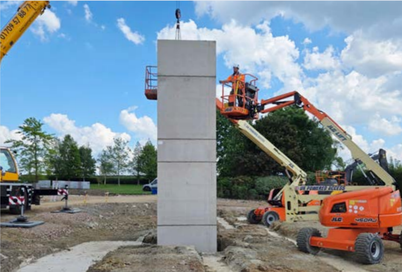
Precast lift shafts enable efficient and safe site working with less formwork, scaffolding and labour.
