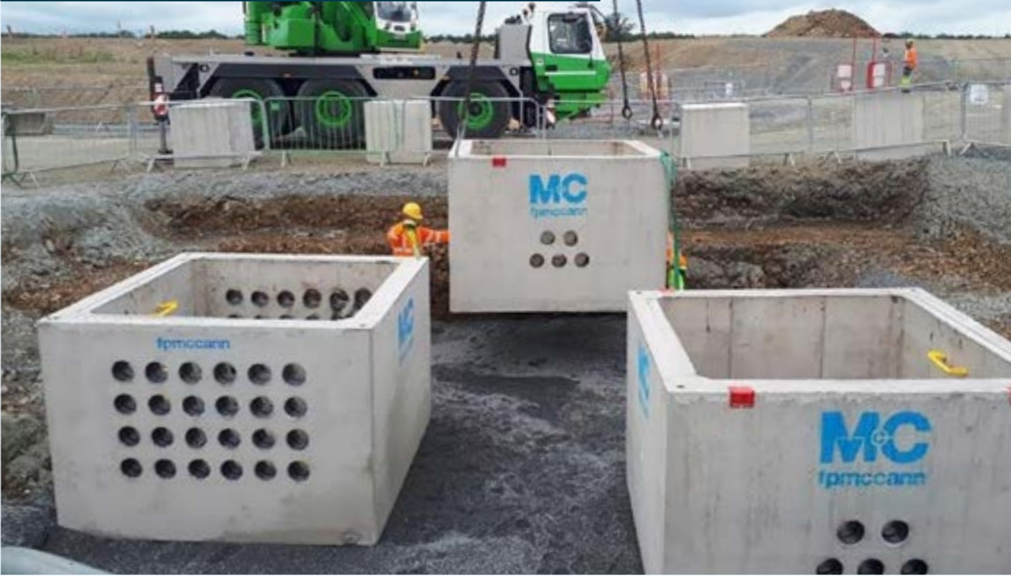
FP McCann’s communication chambers are lifted into position for rapid installation.
