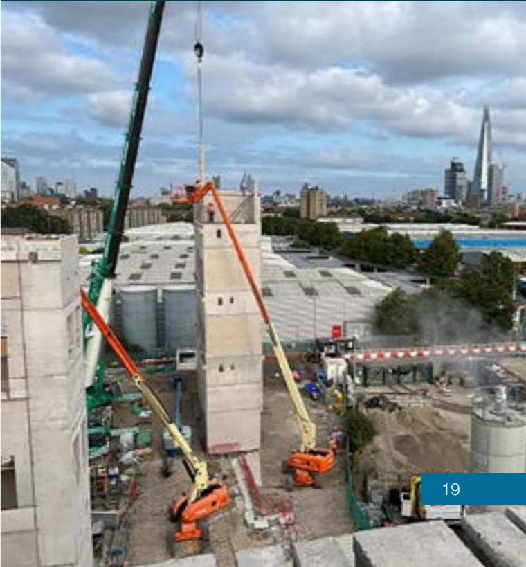
Precast stair cores are formed quickly with low on-site labour demand.
