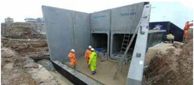
Box culvert with wing walls
