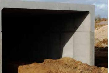
UAN culverts consist of two U-shaped sections, which can then be assembled on-site. A ball and socket joint is used between the two parts of the finished section. This option can be offered for larger box culverts that are unsuitable for transport as a monolithic structure or if there are any site specific weight constraints.
