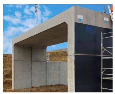
Portal frames either consist up of an n-shaped upper unit and two L-shaped footings per ring, or simply just an n-section. The portal frame system offers a quicker and more economical alternative to bridge beams and abutments that are cast in-situ. Units can be designed for specified loadings, and fulfill Eurocode requirements.
