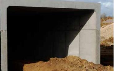
UAN culverts consist of two U-shaped sections, which can then be assembled on-site. A ball and socket joint is used between the two parts of the finished section. This option can be offered for larger box culverts that are unsuitable for transport as a monolithic structure or if there are any site specific weight constraints.
