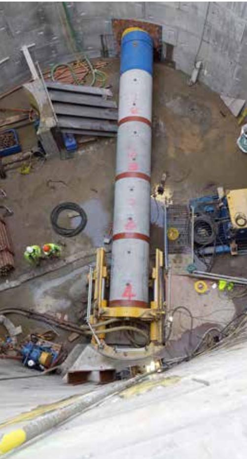
As well as the large 15metre diameter, storage tank capable of holding 1700m<sup>3</sup> of storm water, the project involves four drive/reception shafts, 550metres of DN 1200mm and 70 metres of DN 600mm pipe jacked tunnel, also acting as online storage. FP McCann has supplied both the smoothbore precast concrete shaft segments and the jacking pipes to the contract.
