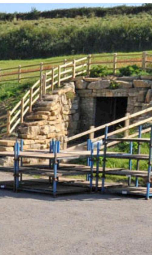
The 'cave' was installed after MJ Fry Engineering had completed substantial groundworks, excavating a hole in the side of a hill that was deep enough to accommodate a 3 metre effective internal wall height, with an additional 3 to 4 metres of soil / backfill on the external top. This was integral to the design, to allow for an additional surcharge load from a light duty tractor which mows the grass on the top of the soil fill.
