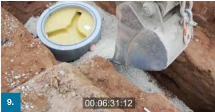
9. Back filling around the connection pipes protects the joint and outlet pipe from damage.
