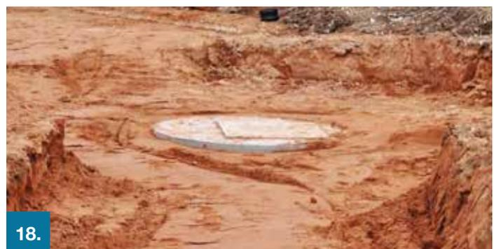
18. From start to completion, most manhole installations using the FP McCann easi-base system will take less than an hour.
