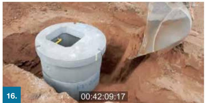
16. In the case of the wide wall manhole chamber ring, the robust design means the requirement for a concrete surround is eliminated.
