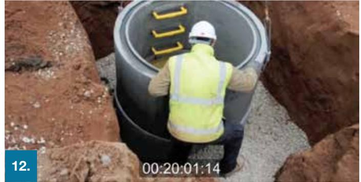
12. The DN1200 easi-base shown can accommodate both standard 90mm thick manhole chamber or as shown the 130mm wide wall manhole chamber ring.
