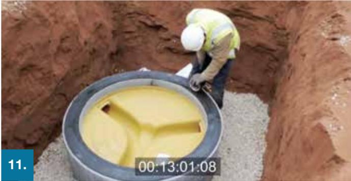
11. Once compressed between jointing faces, the strip will provide a permanent seal. It is important to overlap the sealant strip.
