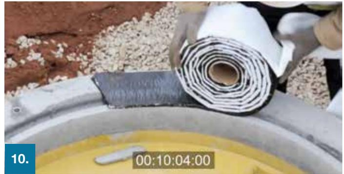
10. Before building on the easi-base with chamber rings, it is recommended the a bitumen sealant strip be used.
